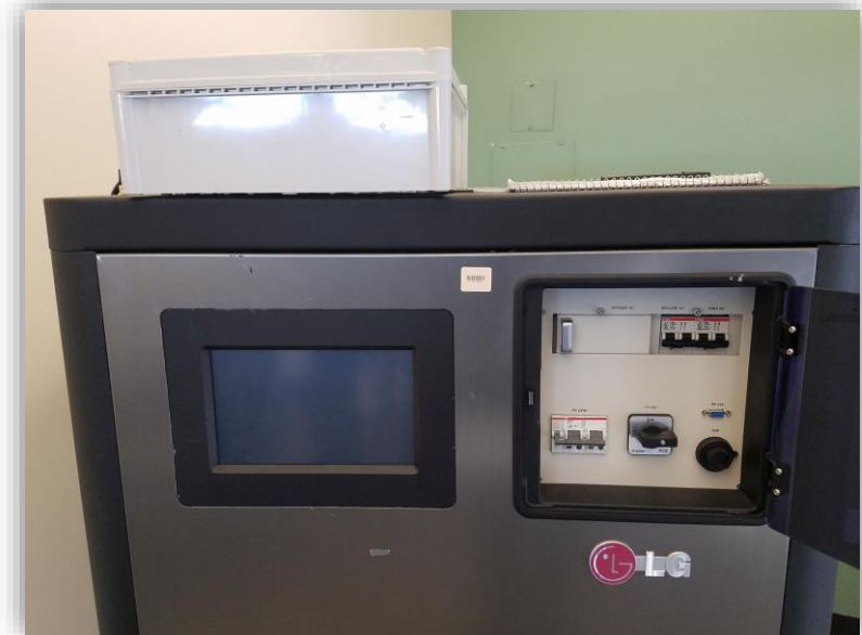
Residential Energy Storage Unit (RESU) block:
